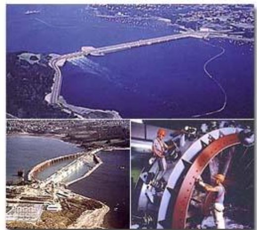
Photo credit: Popular Mechanics , December 1997. Top picture shows water flowing from left to right. Bottom left shows project while under construction. Right picture shows turbine assembly and blades.
